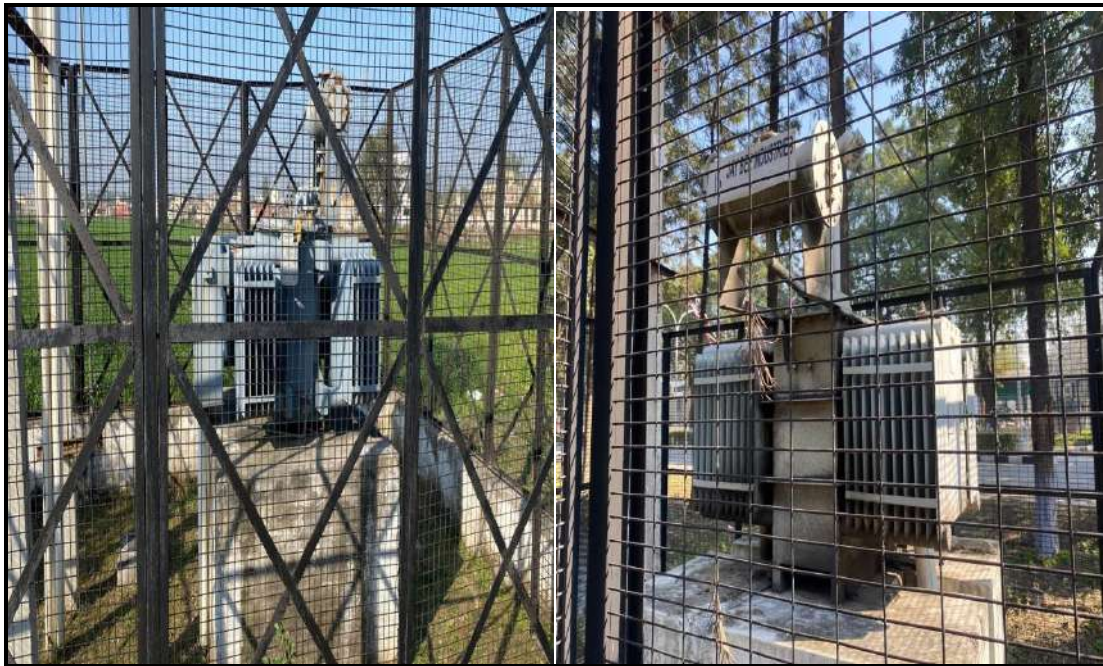
Figure :- Two 315 KVA Transformers – (i) near STP plant and (ii) near Techer club
