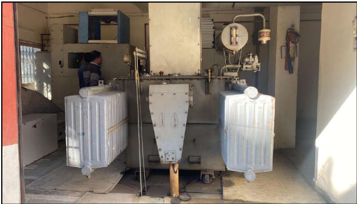
Power House No-4
