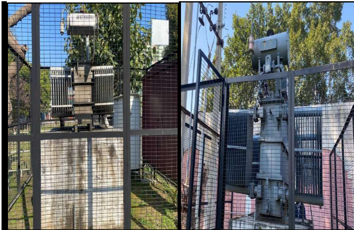
Figure :- (i) 315 kVA TR near UIET Meachanical and (ii) 1000 kVA TR Near University market
