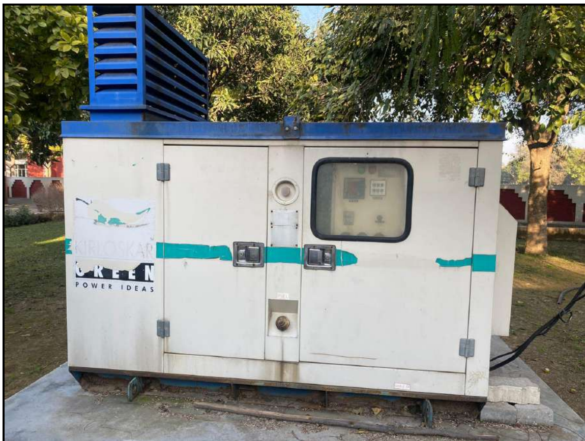
Figure: - DG-sets for Geophysics at KUK
