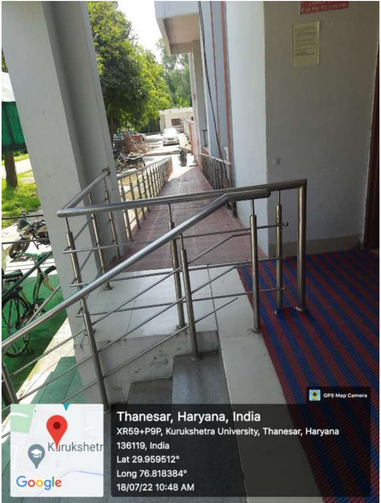
(Ramp at Examination Branch Wingh-II)
