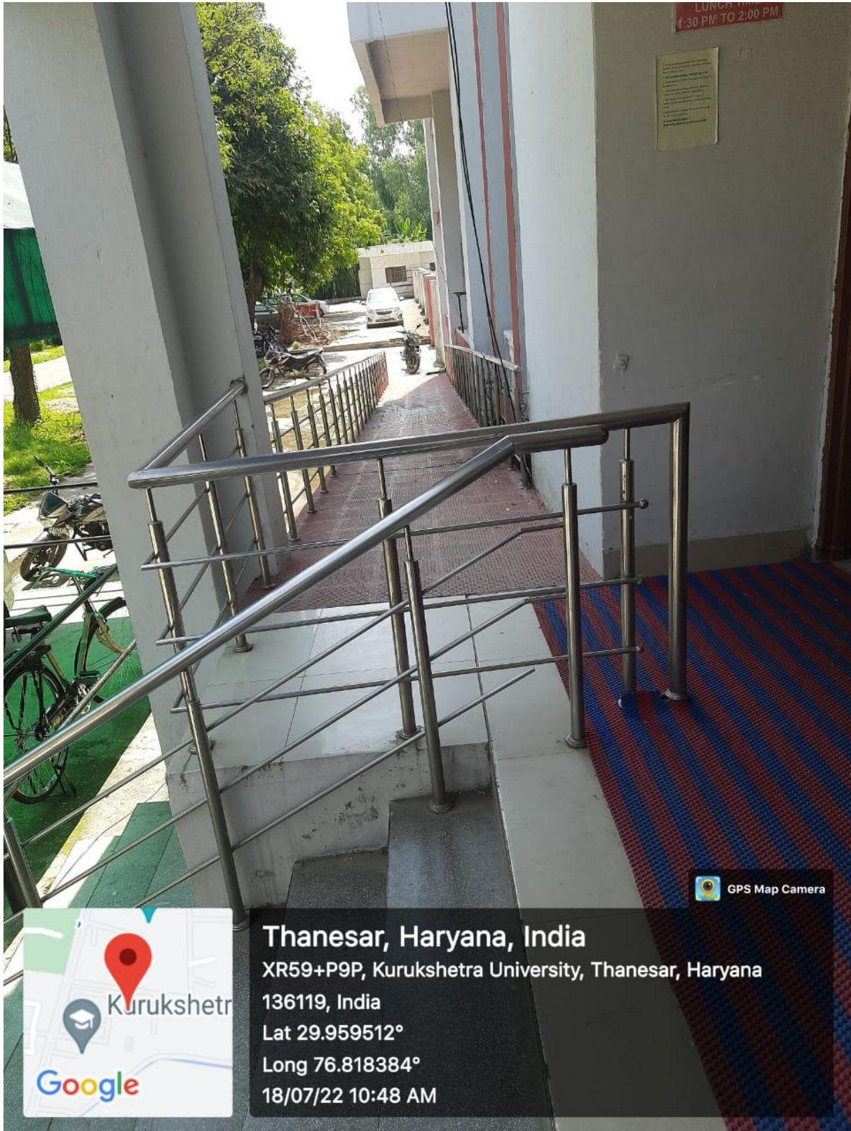
(Ramp at Examination Branch Wing-II)
