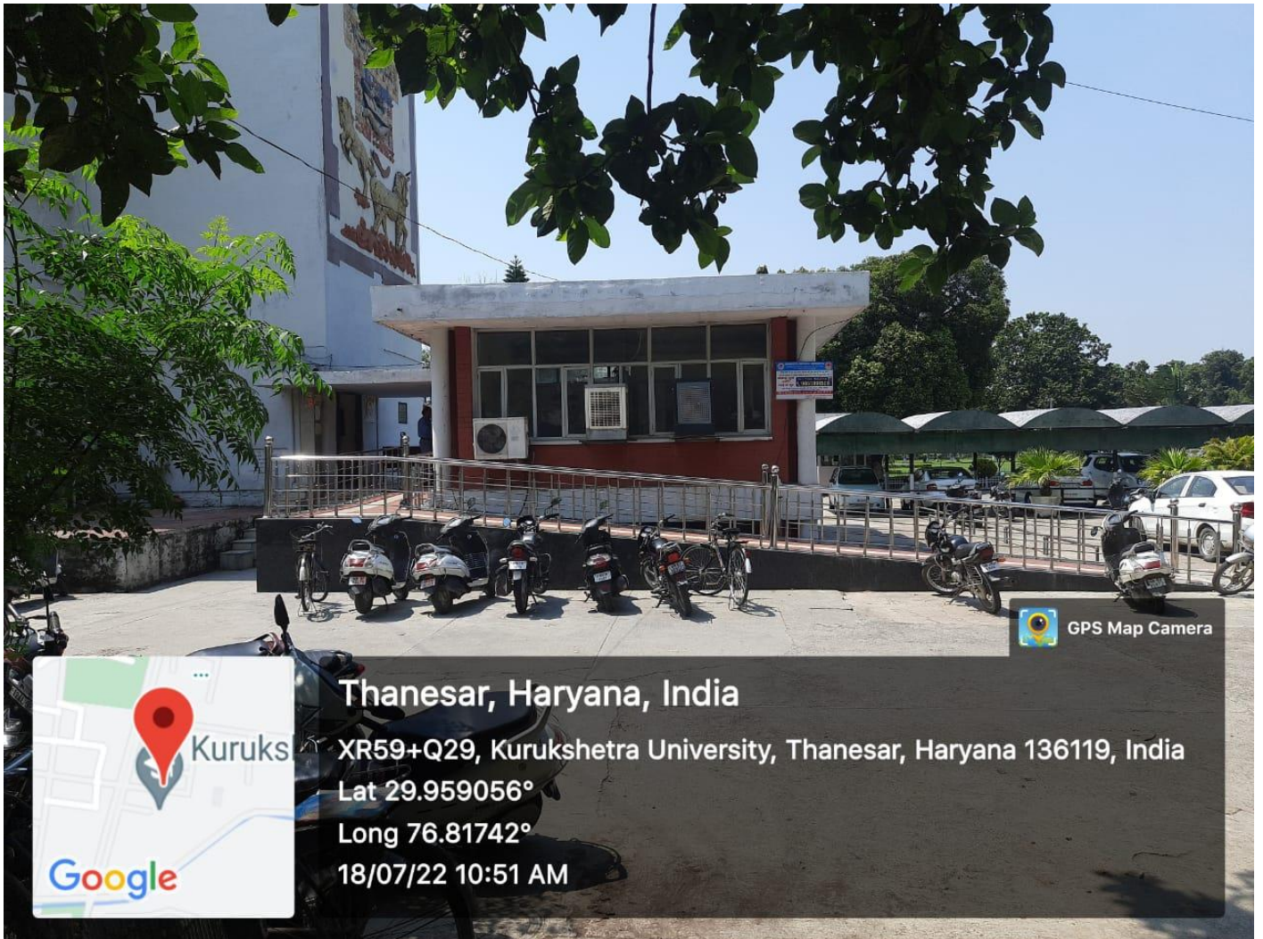
(Ramp at Administrative Block)
